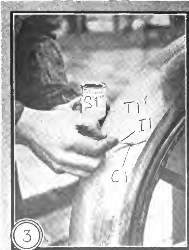
STEP BY STEP IN THE PROCESS OF REPAIRING TIRES AND CASES, BEGINNING WITH THE EXAMINATION AND CLEANING.
